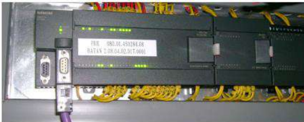
FIGURE 3. Main controller of the safety system using the S7-200 PLC.
