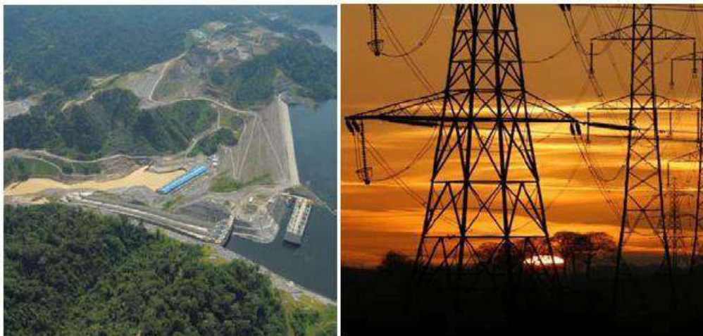
GAMBAR 1. Bakun Dam Hydro Electric Power (HEP) 2400 MW.
